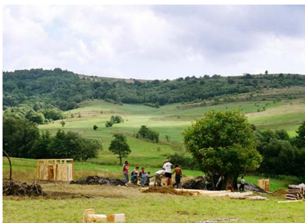
Building the Dungo Spa Community Baths in 2006. Photo: Anna Varga
